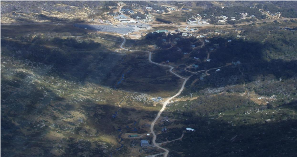
Figure 22i. Perisher ski resort is built adjacent to extensive subalpine shrub bogs and has placed structures, car parks and drainage works on some areas of mire. April 2004. Photo: Geoff Hope
