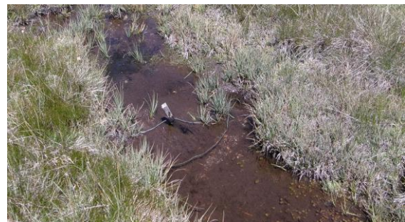
Figure 22c. Sterilised straw bale impeding drainage, Valentine River, February 2010. Photo: Genevieve Wright
