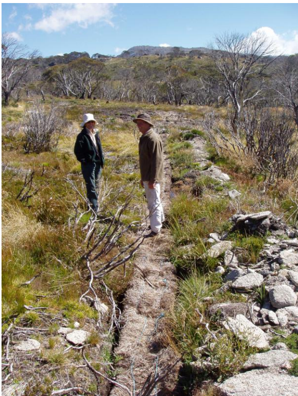
Figure 22b. Amanda Carey and Roger Good examining a straw bale barrier placed in a ditch, April 2005. Photo: Trish MacDonald
